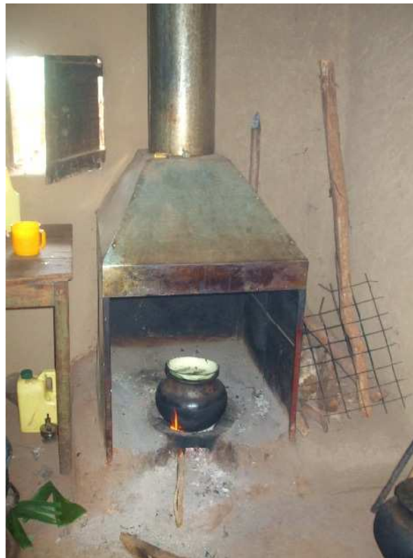
Figure 5.7: The smoke hood
