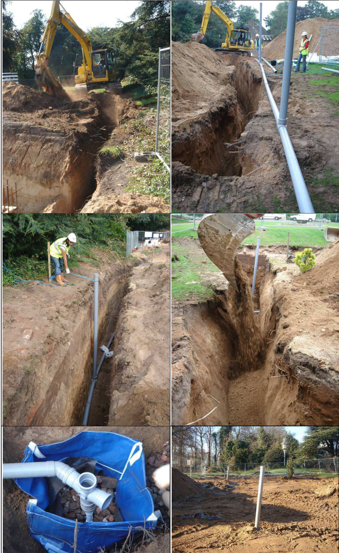
Figure 6-18: The construction of the Stoneguard House EAHE
