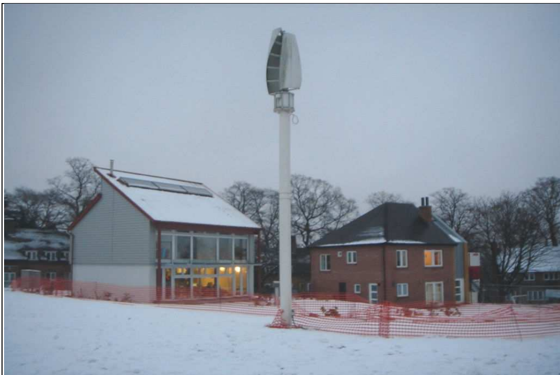
Figure 7-1: The BASF House (left) next to its neighbour, the Eon House, built to 1930s standards (uninsulated) 67 . The BASF House is highly insulated so little heat escaped by conduction through the roof allowing snow to settle.
