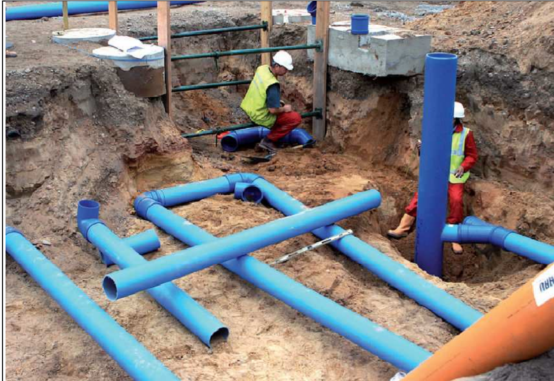
Figure 7-16: The installation of the Awadukt EAHE in the BASF house plot
