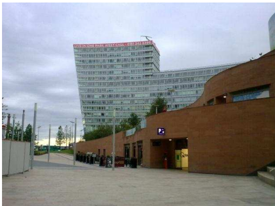
Figure 5.17. The wavy mass at the original edge of the Old Wet Dock emphasises the feeling of water, especially with the ship-like Cesar Pelli's One Park West Building in the background
