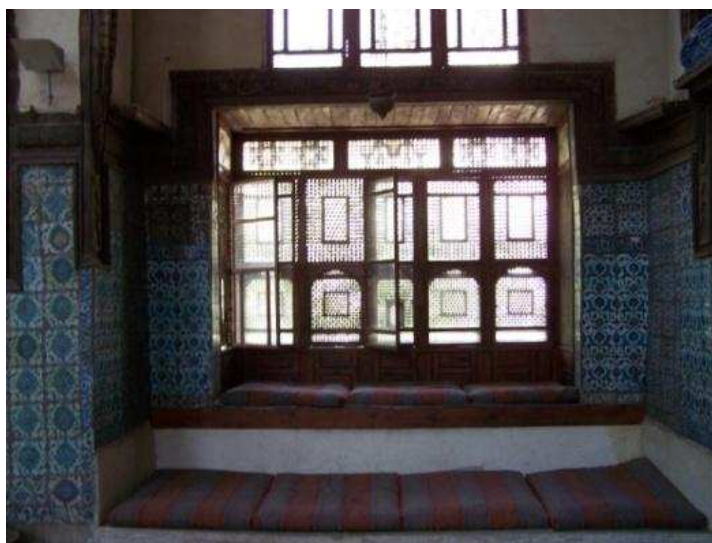
Figure 6. 24. The use of mashrabyya as an ecological treatment for providing shaded-interior with a breath-in in the hot summer days of Cairo- Suhaimy House
