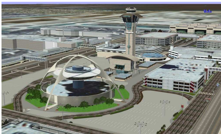
Figure 2.3 LAX Original Condition (UST, 1998)
