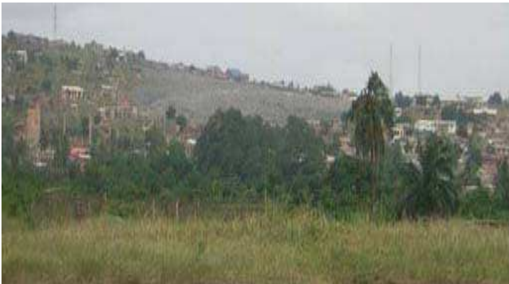
Figure 5.16: The landfill at Oblogo, located close to residential areas
