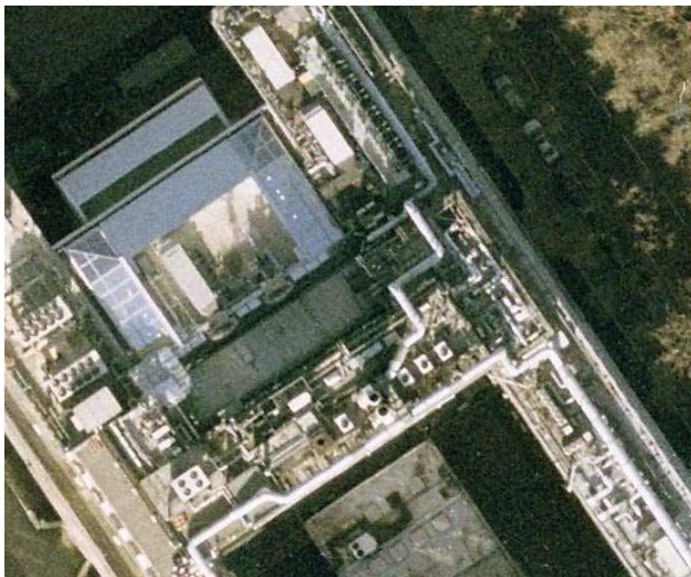
Figure 67. Example of complex building roof geometry present in the second study area
