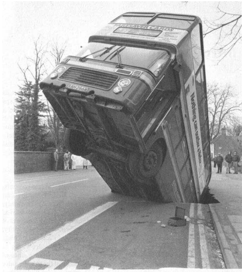
Figure 1.1 An example of (extreme) subsidence. Road collapsed beneath a bus, due to failure of weathered chalk above an abandoned mine, in Norwich, U.K. ( Waltham 1989 )
