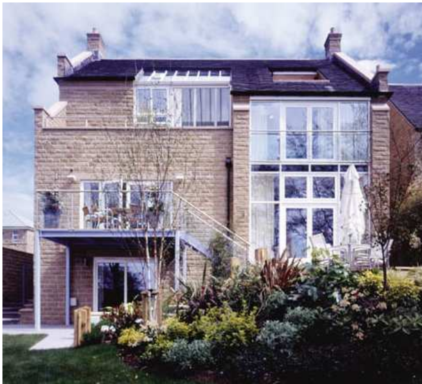
Figure 8: The vernacularly styled front and heavily glazed rear elevations
