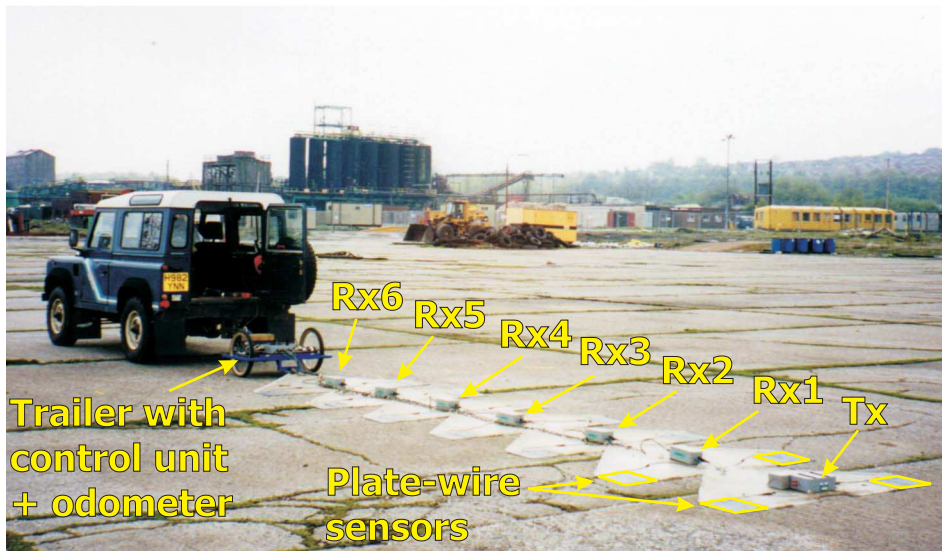
Figure 7.14: The CORIM™ system in field operation.
