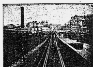
APPROACHING THE BROOKLYN TERMINAL.
