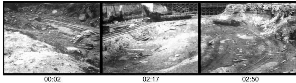
Fig. 5.6 Frames from Pennsylvania Tunnel Excavation (AM&B, 1905).
