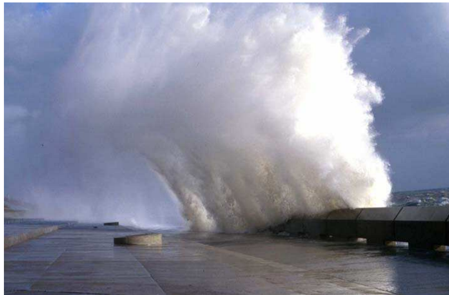
Figure 1.1: Severe wave overtopping at the Samphire Hoe seawall, UK (from CLASH project, www.clash-eu.org (2001)).
