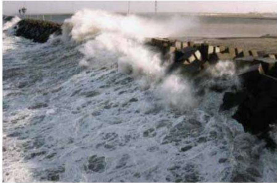
Figure 1.2: Wave run-up and overtopping at Zeebrugge breakwater (Belgium), during (mild) storm conditions (from OPTICREST project, www.rug.ac.be/opticrest (2001)).
