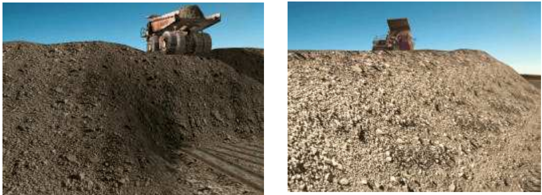
Figure 7-14: Truck falling over edge
