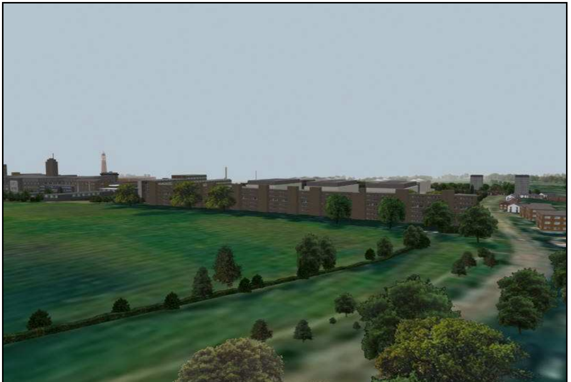
Figure A7.7: Rendered image from critical viewpoint seven showing the proposed hospital 204 .
