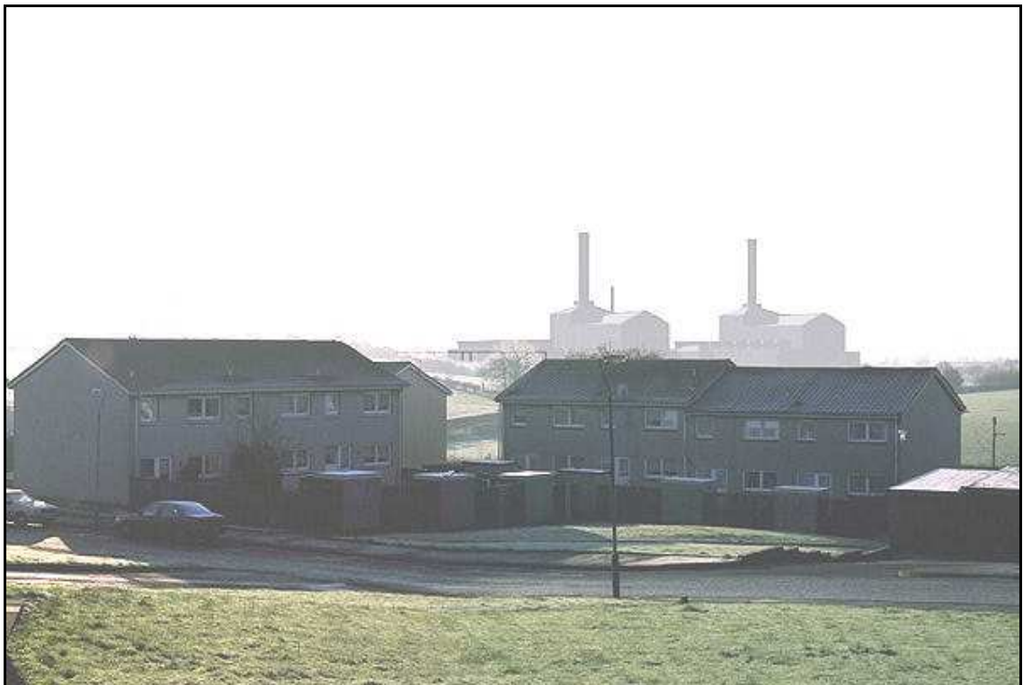
Figure 3.12: A photomontage of a combined-cycle gas turbine power station 50 .
