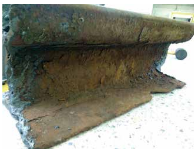
Figure 11. Corrosion affecting the entire length of rail foot and web, rail sample from street-running track
