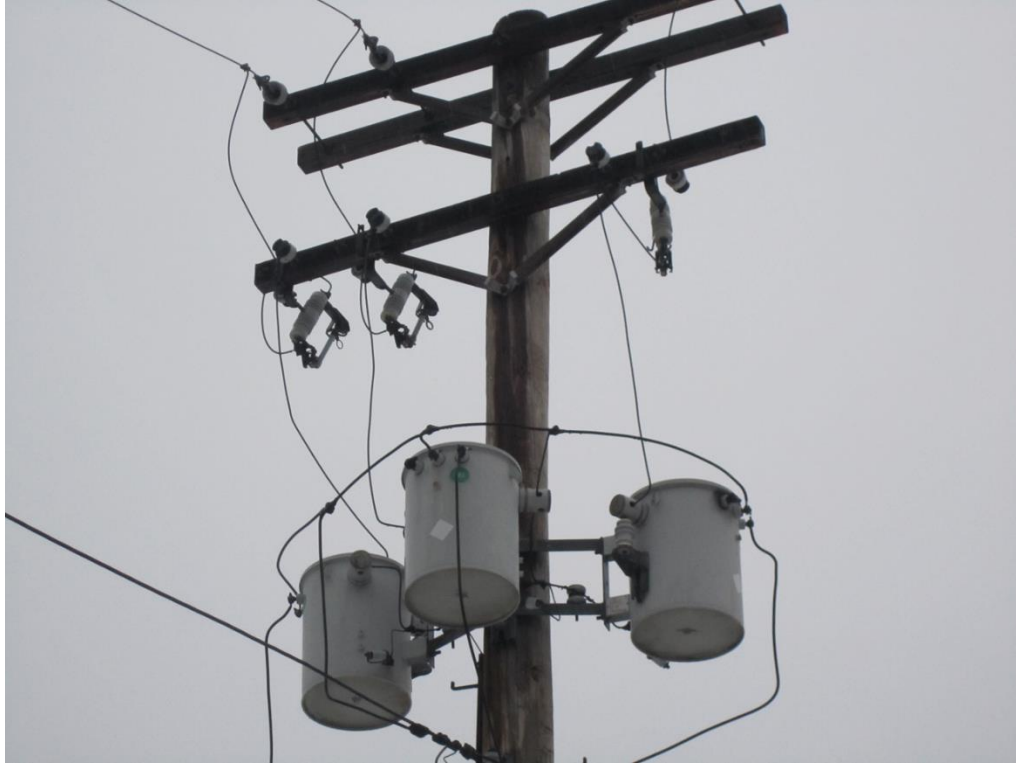
Figure 6 - Distribution primary feeding three-phase secondary
