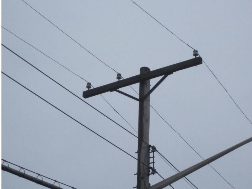
Figure 3 - Distribution three-phase primary
