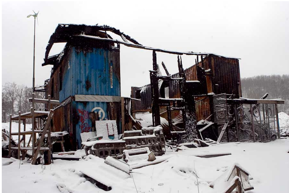
Figure 5-7: Cyklopen after the fire, November 2008
