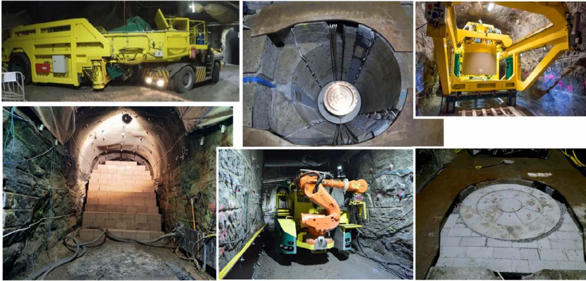
FIGURE L3-3. EBS components installed with prototype machines in FISST.
