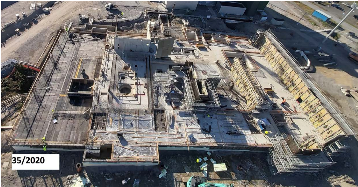
FIGURE L3-5. Construction site of the encapsulation plant.
