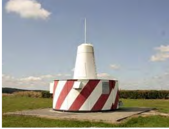
Figure 1.2: A CVOR antenna [wikimedia commons].
