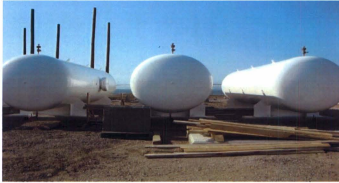
Figure 2.8: Hydrogen Tanks in Ramea
