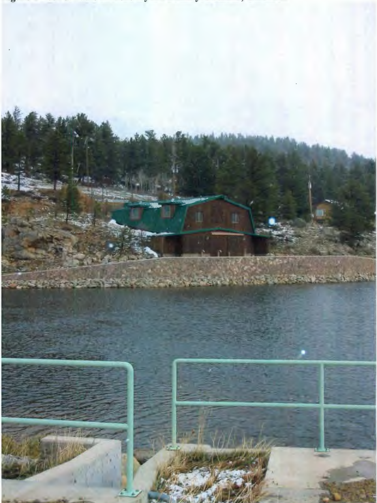
Figure 6 - Silver Lake In-Line Hydro Facility. Boulder, Colorado
