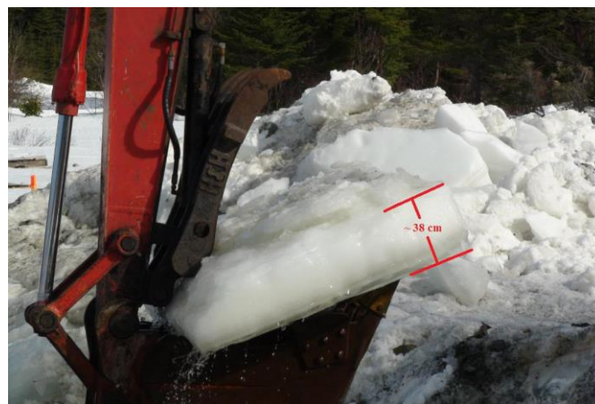
Figure 3.5: Ice floe removal using an excavator
