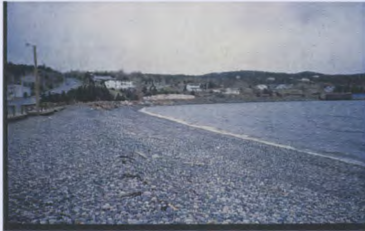
Plate 3.4: The backshore of Holyrood Beach today contains numerous residential and commercial buildings, often constructed very close to the shoreline.
