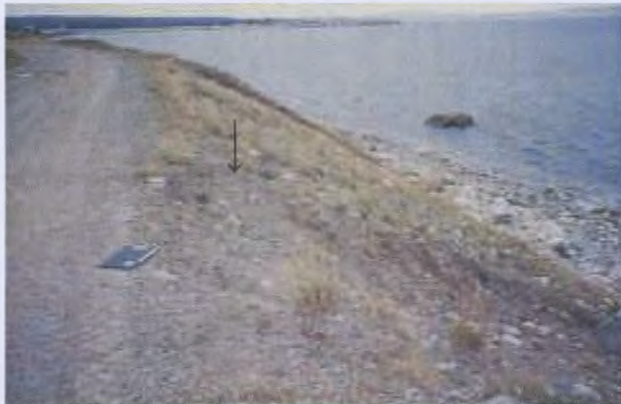
Plate 6.4: Debris flows initiating from the T'railway Recreational trail in Lance Cove (13 225 – 14 203 m).
