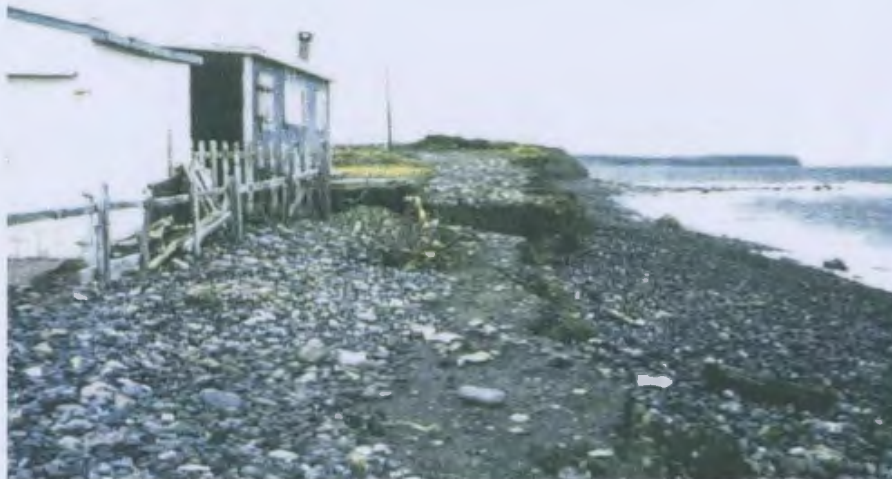
Plate 8.3: Severe erosion to the beach and nearby road following the passage of the October 1992 nor'easter (photograph courtesy Martin Goebel, Department of Environment, Government of Newfoundland and Labrador).
