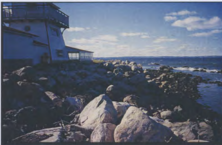
Plate 9.1: This building, adjacent to the Foxtrap Marina (segment 7866 – 7947 m), is located within the 30 m development setback and is less than five metres from the bluff edge. Although the placement of riprap will halt erosion processes, the site can still be impacted by storm waves.
