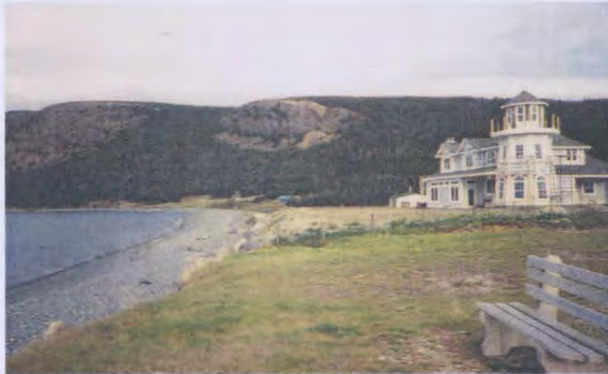
Plate 8.4: New home in Topsail (segment 679 – 759 m) constructed within a coastal hazard area.
