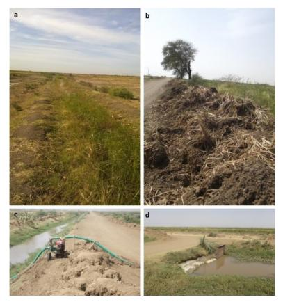
**Fig. S5.2.** Problems in the irrigation canals in the Gezira Scheme: (a) weeds, (b) siltation, (c) improper maintenance resulted in different levels in the canals and (d) broken water gates.
