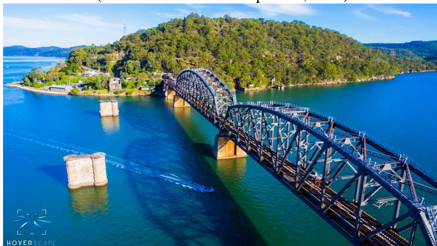
Gambar XLII : Hawkesbury River Railway Bridge (Sumber: www.hoverscape.com , 2015)
