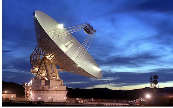
Figure 2.4: A parabolic 70 m dish antenna is used in the Goldstone Observatory station, Mojave Desert, California, USA [4].
