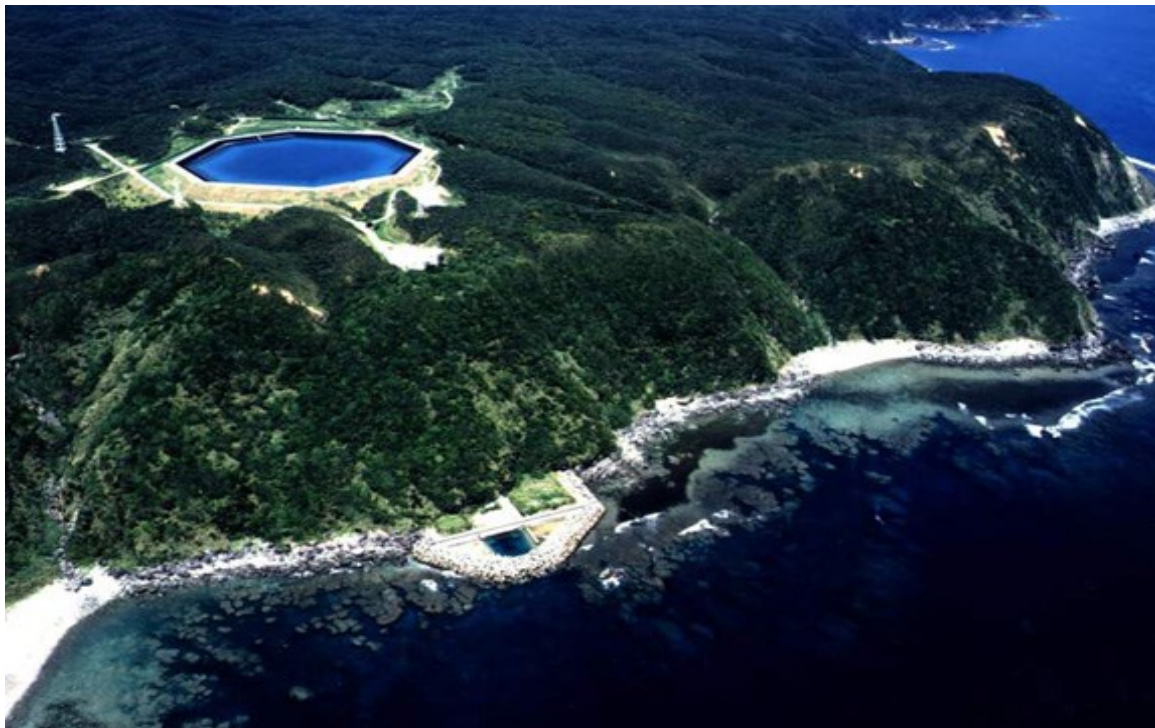
Figure 2: Okinawa pumped-storage power plant, whose lower reservoir is the ocean with 0.2GWh energy stored, source iea hydro power (2013)
