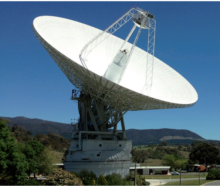
Figure 24. DSS-43 dish at the Canberra Deep Space Communication Complex (CDSCC): a Cassegrain antenna whose diameter is 70 m (image courtesy of NASA).
