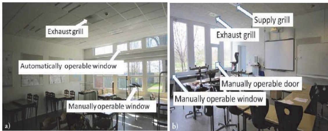
Figure 4. Denmark study classrooms: (a) classroom with automatically operable windows and exhaust fan; (b) mechanically ventilated classroom [31].
