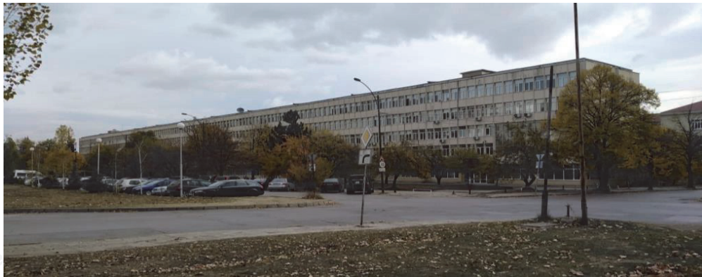
Figure 15. Building 2 of TU-Sofia.
