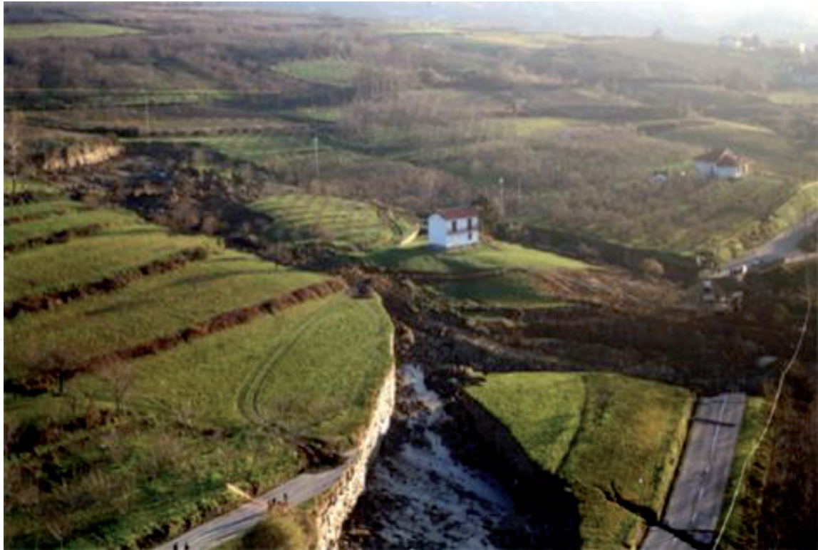
Figure 11. Rock-block slide near Feisoglio town: The mass movement slid about 50–60 m from their original position, destroying a road. The estimated area was about 4.63 ha, while the volume was about 385,000 m 3 . The gray layer surface is evident. The small white house moved together with the rock block nearly undamaged.
