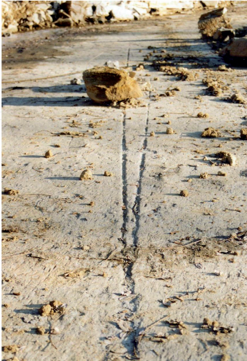
Figure 8. Sliding surface of the Murazzano landslide taken from uphill: The shallow tracks left by the sliding rock blocks are evident.
