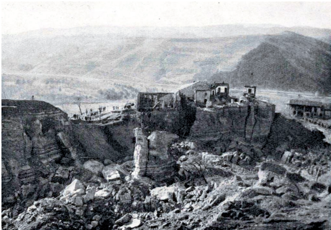
Figure 3. Cissonone, Cascina Bric farmhouse. The large rock-block slide that caused three casualties on April 7, 1941.
