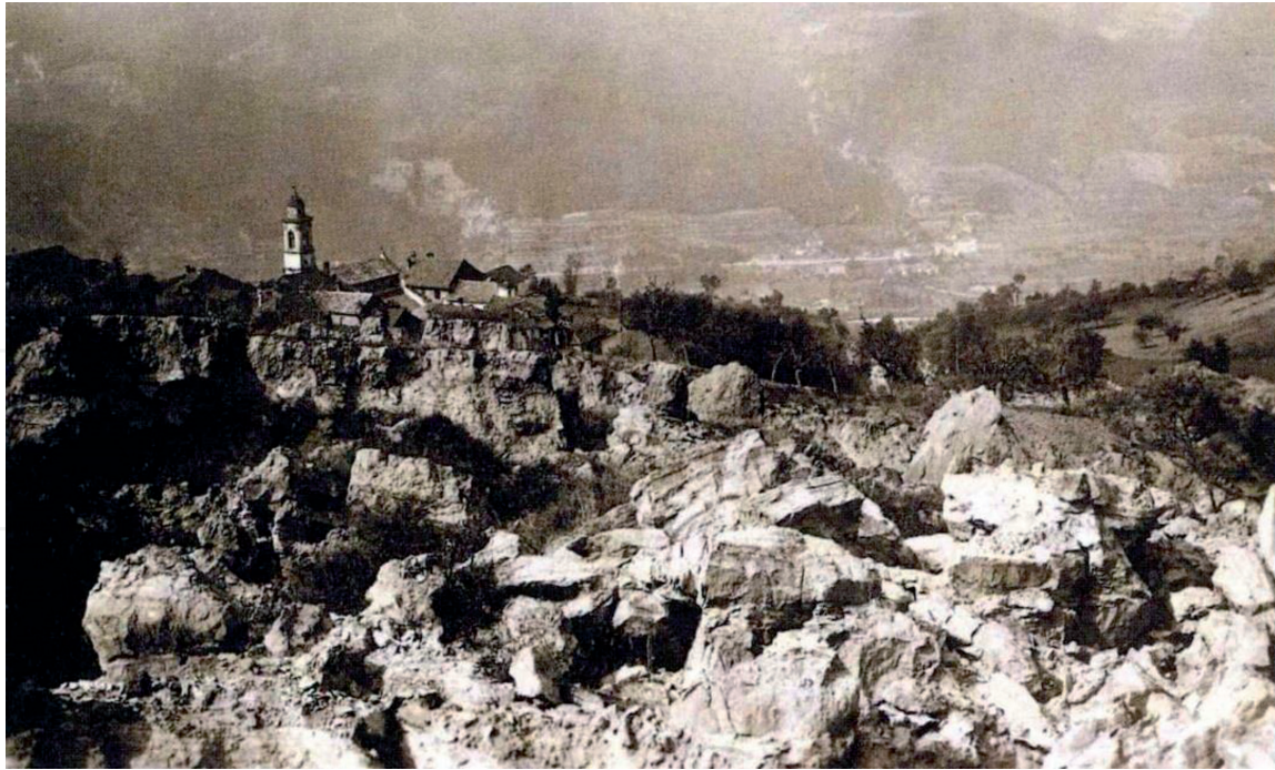
Figure 2. May 16, 1926: Levico rock-block slides, top view. The large disjointed clods are evident.
