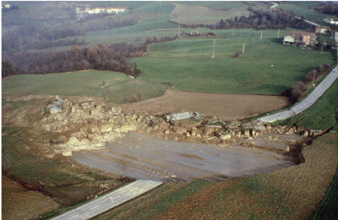
Figure 17. Murazzano rock-block slide, one of the most showy TRBSs triggered in November 1994, here shot a week later when a temporary road had already been restored. The clods moved along a surface with a gradient of 9.8^\circ for a distance of about 80–100 m. The crown was located about 20–25 m upstream of the provincial road.
