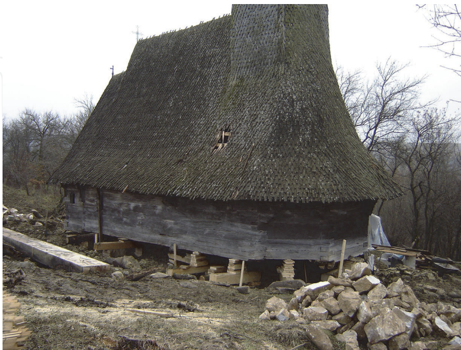
Figure 5. The lifting of the church.
