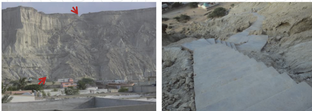
Figure 2. Pedestrian tsunami evacuation route at Gwadar City, Baluchistan Province. (Left) Red arrows show starting and ending point of the evacuation route. (Right) Tsunami evacuation route, more than 600 steps of a stairs designed with landing at several points to facilitate pedestrian evacuation leading to the proposed evacuation site at the top of the Koh-e-Batil (a 450 high mountain) by the district disaster management authority Gwadar. Photo by Ghazala Naeem.
