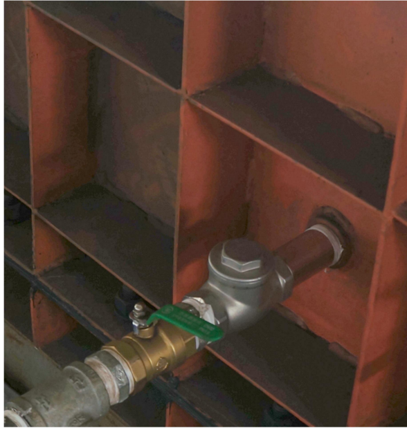
Figure 6-15: One-way valve
