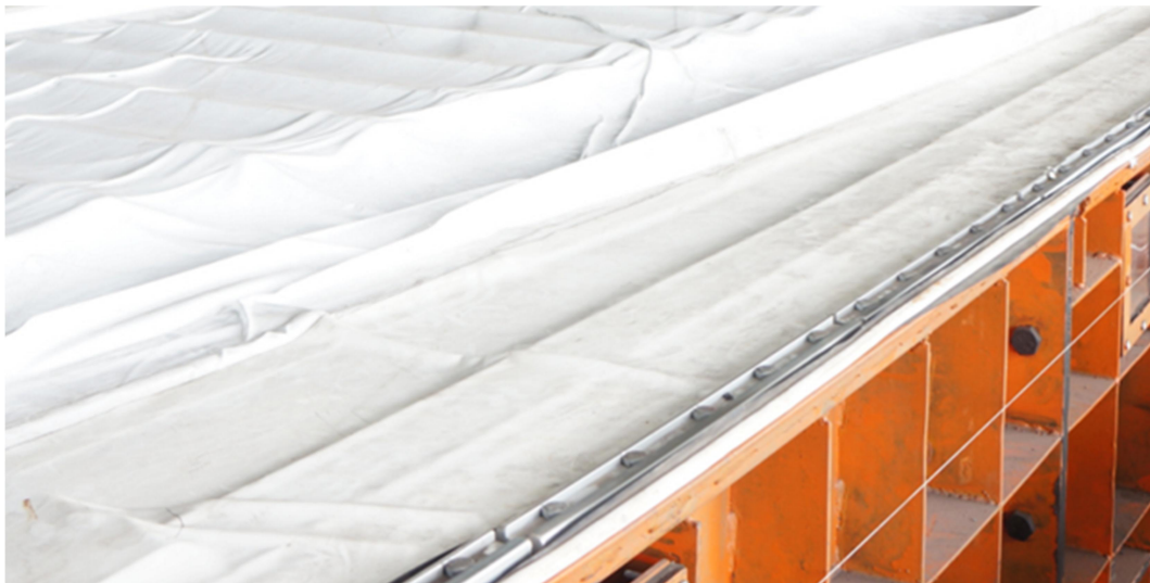
Figure 6-14: Membrane to chamber connection
