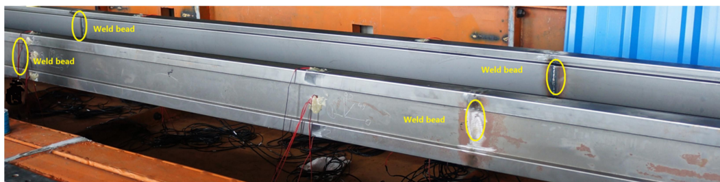
Figure 6-11: The purlin with weld beads
