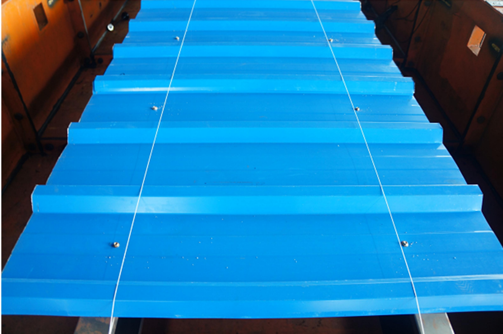
(a) Sheets to purlin connection
