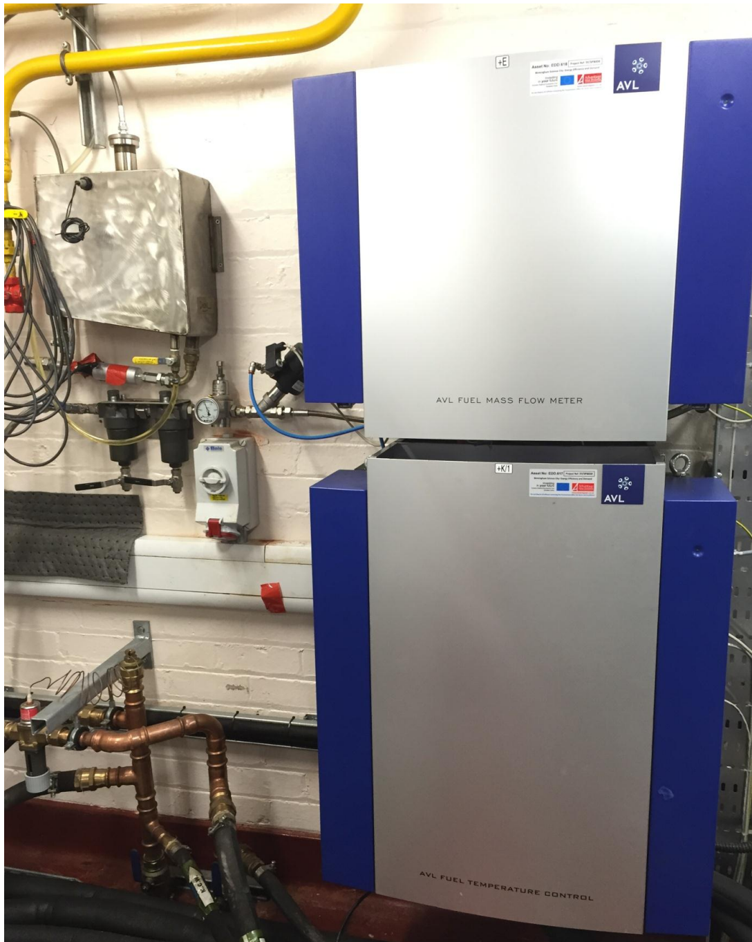
Figure 3-6 Arrangement of Fuel Conditioning System
