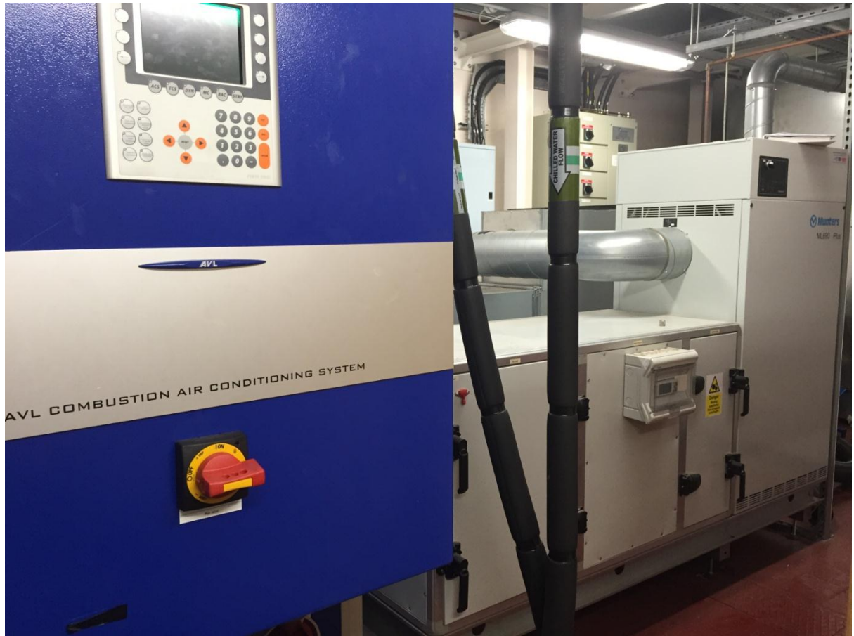
Figure 3-8 Engine Combustion Air Conditioning System
