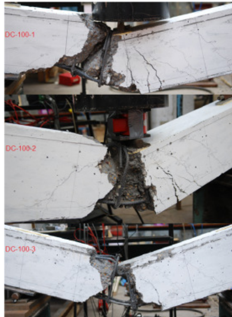
Figure 6.15: Failure modes for DC-100 beams
