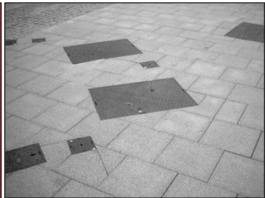
Figure 4-5: Pavement with high quality finish in Eastside (Jefferson et al., 2006)
