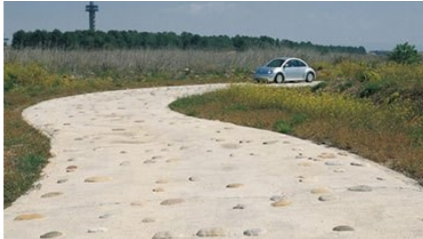
Figure 2.7: A Cobblestone Road in IDIADA
