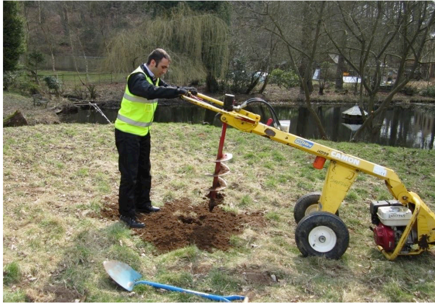
Figure 6.7 Hydraulic posthole borer used at location "A"
