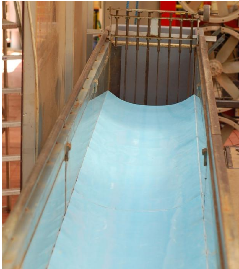
Figure 34. The 1 mm PVC layer was replaced by a 2mm layer, reducing the undulation.
