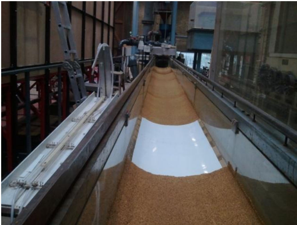
Figure 38. First, glue was applied over a PVC layer, later the section was filled with sand. At the following morning, the excess of sand was removed.
