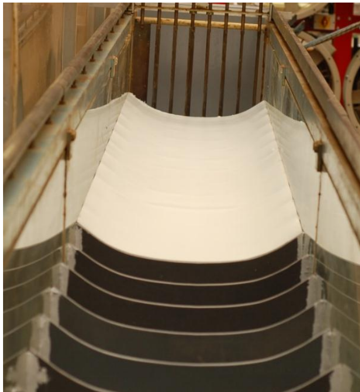
Figure 33. A PVC layer of 1mm was placed over the supports, showing a high undulation between them.
