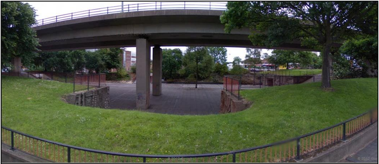
Figure 20: Hockley flyover (Source: Google Streetview)
