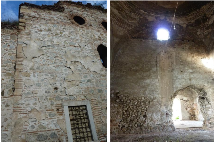
Pl. 48: Koca Mustafa mosque (late 15th c.): a) exterior surface of kibla wall showing the difference in building phases, b) view of the western wall of the principal building phase allowing to western tabhane (Photo: Bessi 2010)
