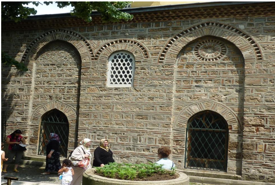
Pl. 14: Puşinpuş Zaviye at Yenişehir south- eastern view (Photo: Bessi 2012)
