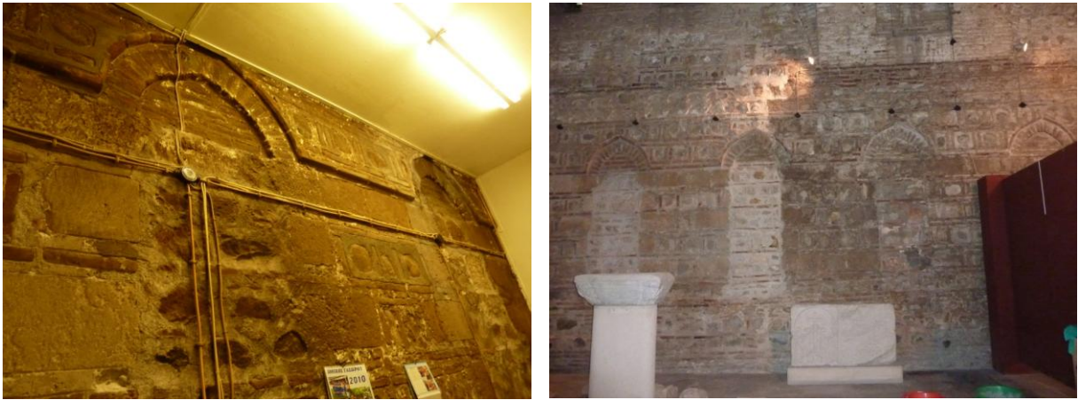
Pl. 65 a-b. Siroz bedesten : blocked windows of the principal building phase (Photo: Bessi 2010)
