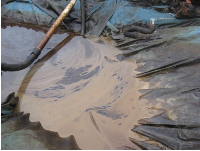
Figure 4.2: Sludge on Swansea site.
