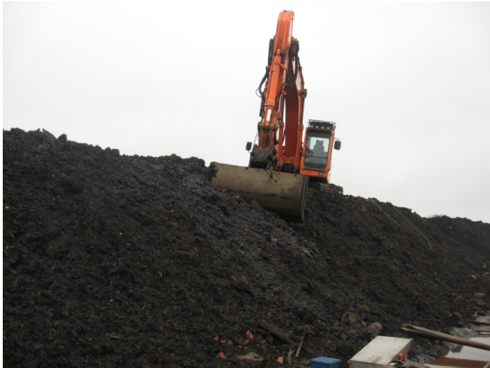
Figure 4.1: Tractor mixing soils on biopiles to facilitate aeration.
