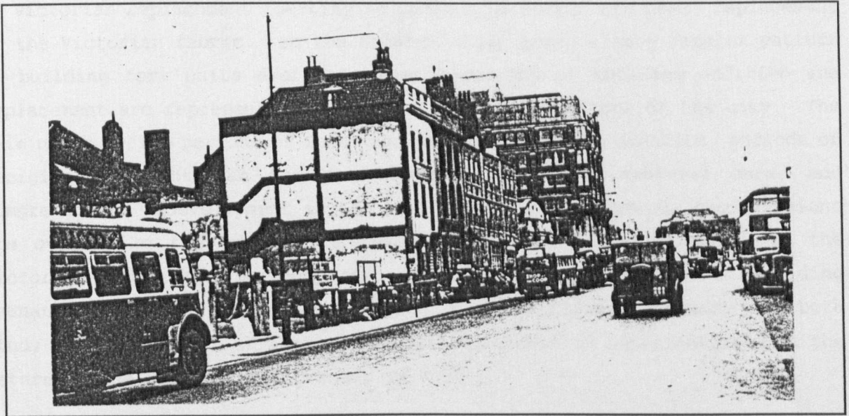
Figure 4.22; Prince Street c1952 showing the remnant Georgian fabric prior to redevelopment as Narrow Quay House and the Unicorn Hotel (source, Bristol CC planning files).
