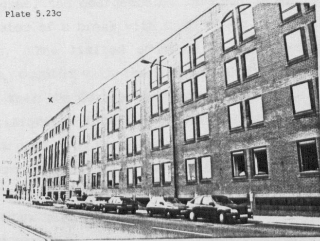
43-45 Queen Square, Bristol (elevation to The Grove)
