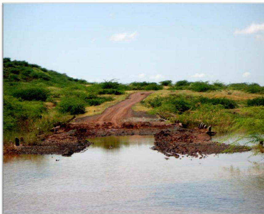
Plate 9-4 The 30km length narrow road connecting the village to the Taluka broken and drowned during monsoon ( source: author, Oct, 2011 )
