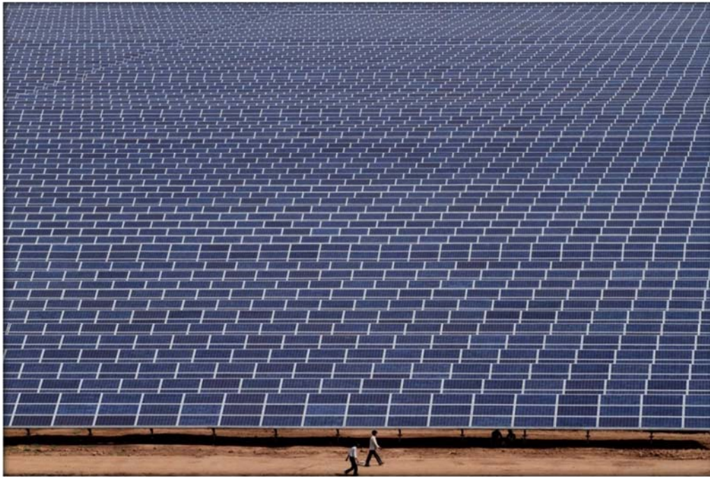
Plate 6-1 Gujarat solar park after commissioning ( Source: Gujarat Solar Park, April 2012 )
