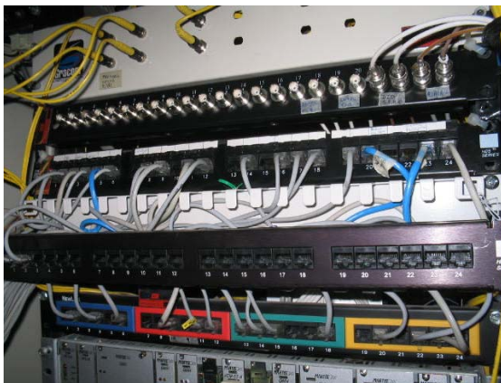
Figura 13. Patch panel
