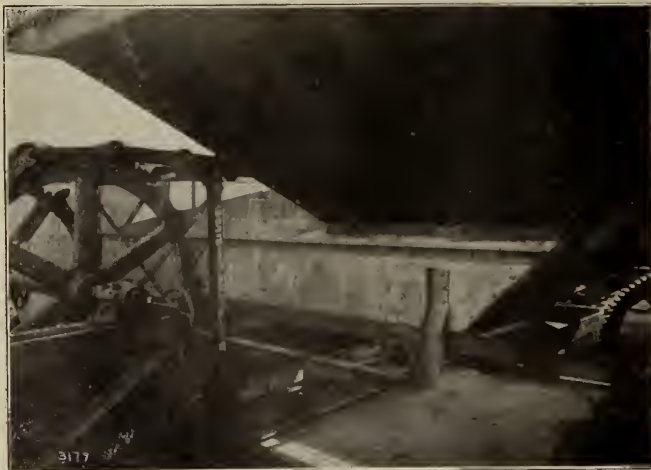
FIG. 4—LOCOMOTIVE COALING STATION, SHOWING TRACK HOPPER WITH RECIPROCATING PLATE.
