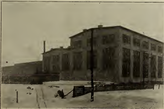
Machine and Erecting Shop, Stratford, Ont.
