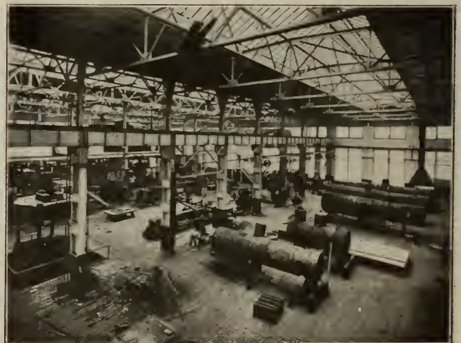
Boiler Shop, Battle Creek.
