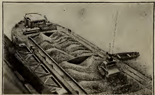
Fig. 3. Looking at Loaded Barge from Operator's Booth.
