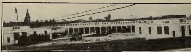
New Round House at Richmond, Cal.
