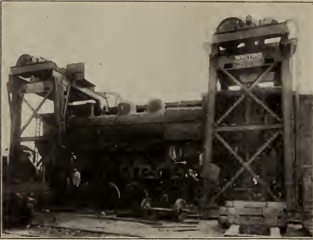
ELECTRIC GANTRY CRANE.
