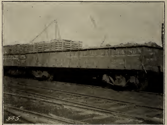
Car Painted with Silica-Graphite Paint After Eighteen Months' Service.
