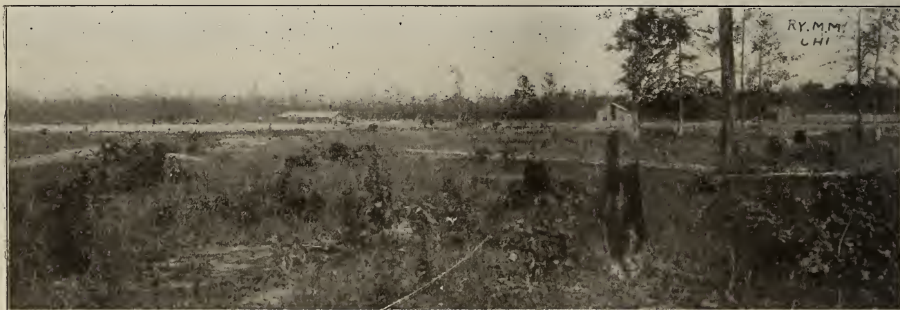
View Showing Nature of Ground on Shop Site
