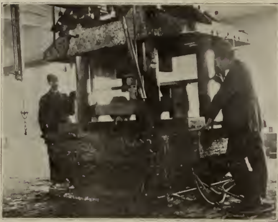
FIG. 6—GAUGING TO FIND IF TRUCK IS STRAIGHTENED TRANSVERSELY.
