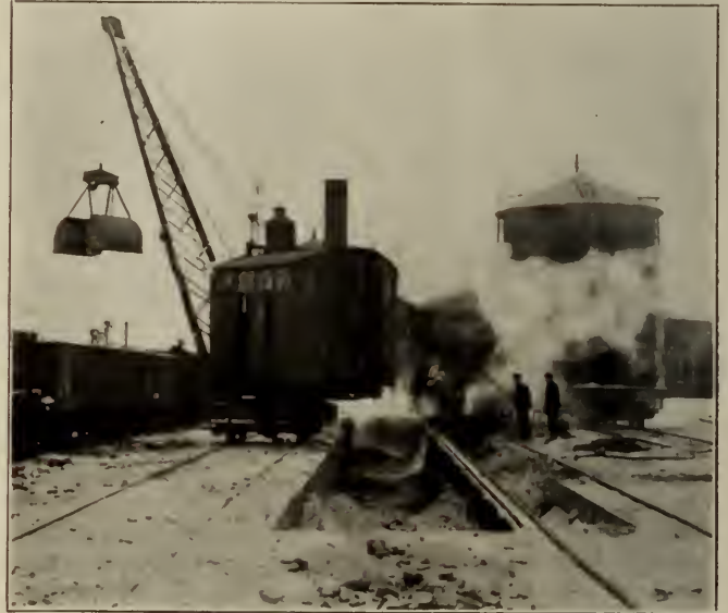
Fig. 2—Locomotive Crane, Nickel Plate Railroad.
