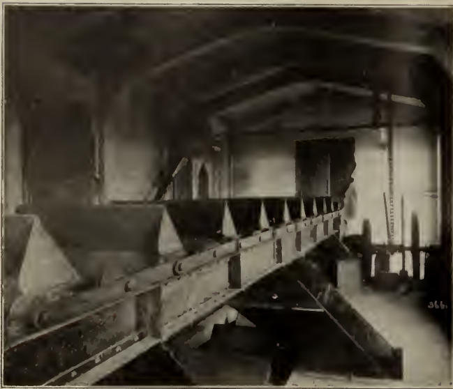
FIG. 3—LOCOMOTIVE COALING STATION, SHOWING V-SHAPED STEEL BUCKETS.
