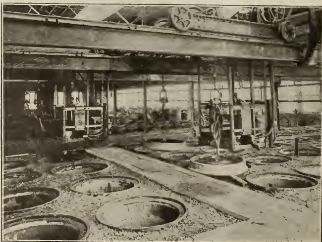
Wheel Pits with 2-Motor Electric Pitting Trolleys.
