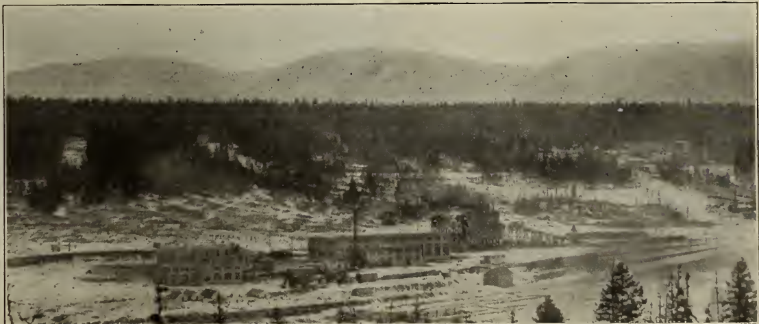
Birdseye View, Idaho & Washington Northern Railroad Shops.
