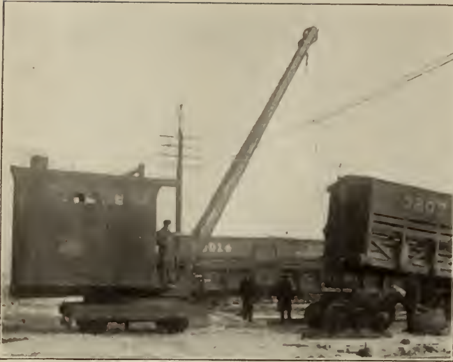
Fig. 1—Locomotive Crane, Car Repair Work.
