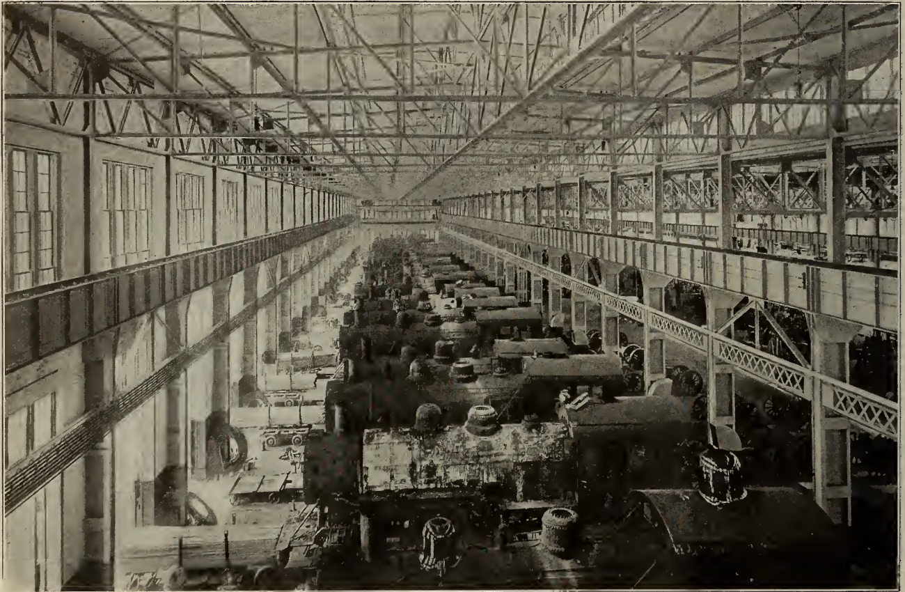
Pit Bay of Erecting Shop, Springfield Shops.
