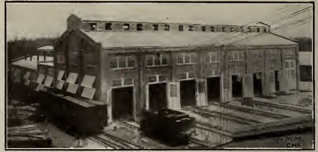
Exterior of Erecting Shop
