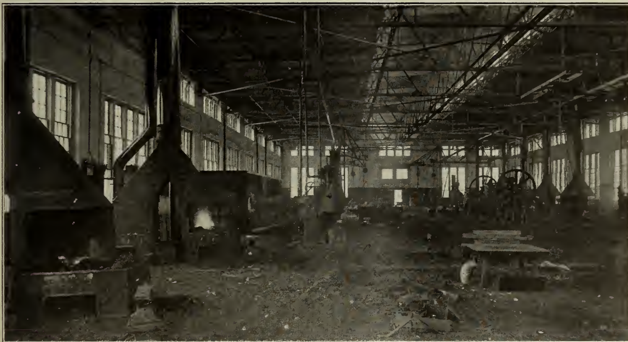
General Interior View of Blacksmith Shop, Springfield Shops.
