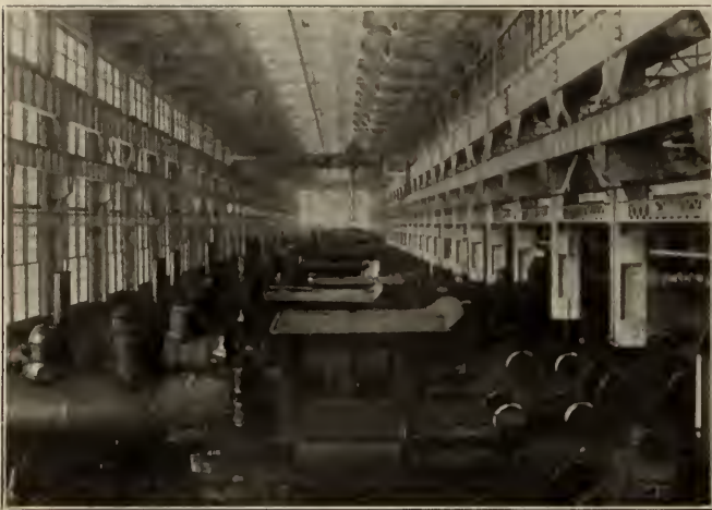
Erecting Shop, Stratford, Ont.
