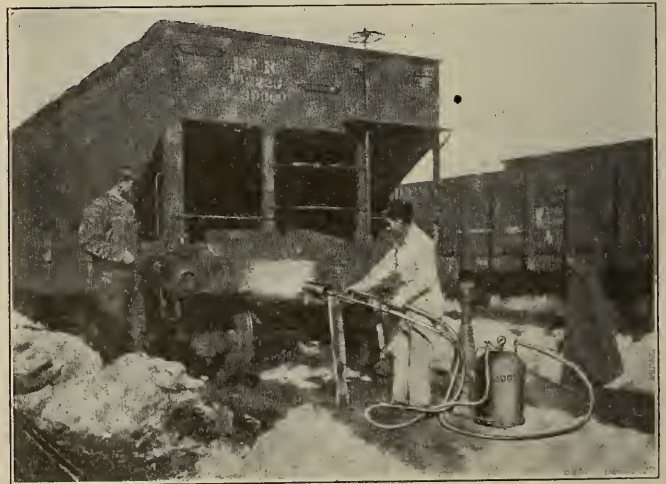
Repairing Steel Car Plates with Burner.
