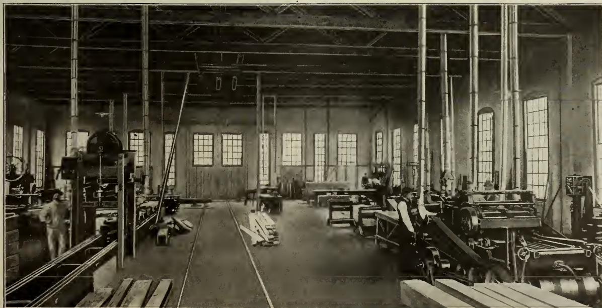
General View of Planing Mill, Boulton Shops.
