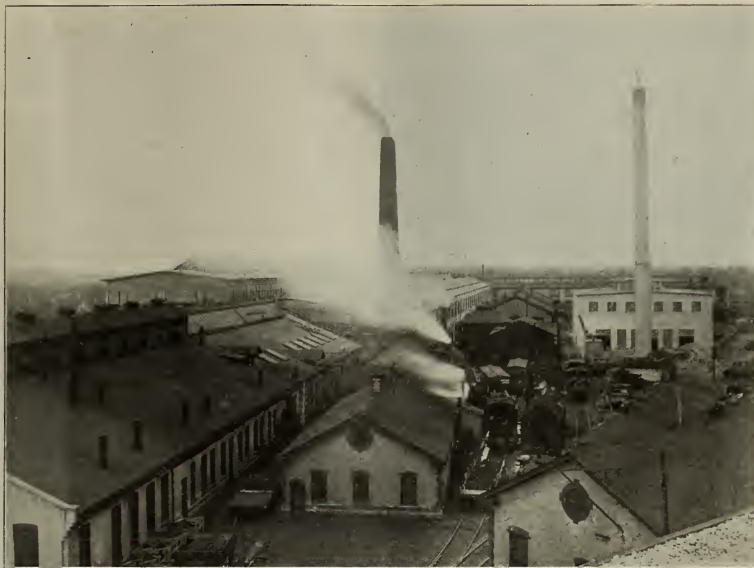
View of Locomotive Repair Shops, Stratford, Ont.
