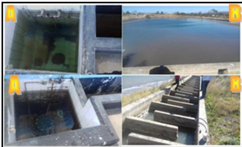
Figure 8.16 – Facilities used at Alice (A) and Fort Beaufort (B) Water Work
