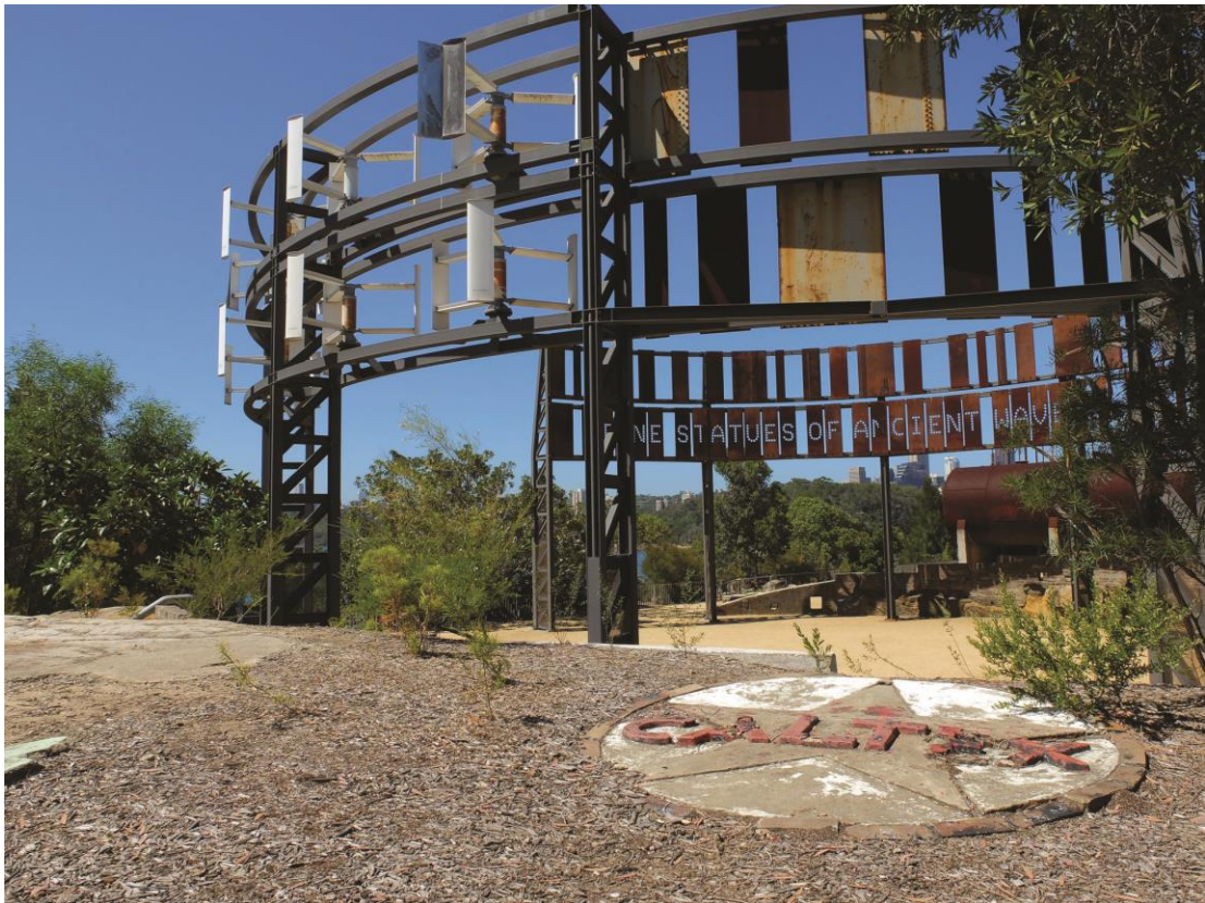
Figure 6.6. Renewable Energy Sculpture: Micro wind turbines integrated into the structure built with recycled material from the former Tank101 once was standing at the same location. Image by the author.
