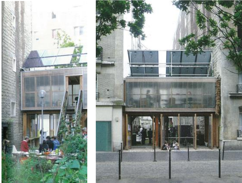
Figure 2.6. Views of ‘Passage 56’ by Atelier D’architecture Autogeree-AAA (Rambert, 2010).
