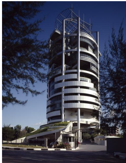
Figure 2.2. Mesiniaga Tower by Ken Yeang, Malaysia (Couzens, 2012).
