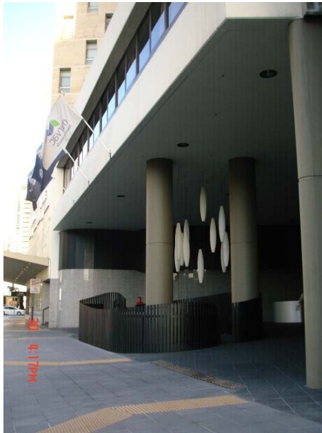
Figure 4.40: Building in (Text)/Building exterior in relation to interior from stage one participant.
