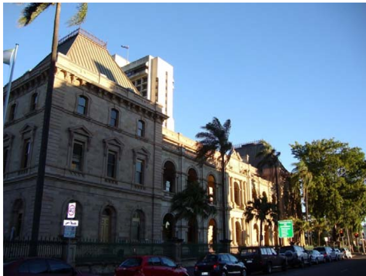
Figure 4.48: Building in (Text)/Building façade and façade elements in relationship from stage one participant.
