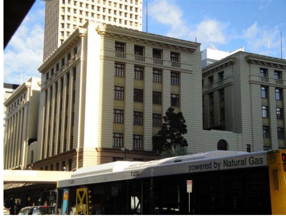
Figure 4.53: Building in (Text)/Building façade and façade elements in relationship from stage one participant.
