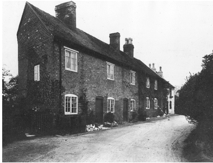
18. The Royal Oak (white at far end) and Royal Oak Cottages, taken by Police Sergeant Moore before 1916. The road was not paved.
